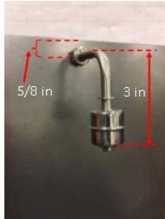
Figure 5b View from inside tank
